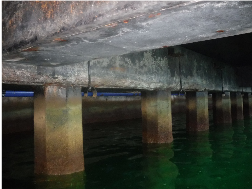
Photo 2: Typical Pier Substructure
